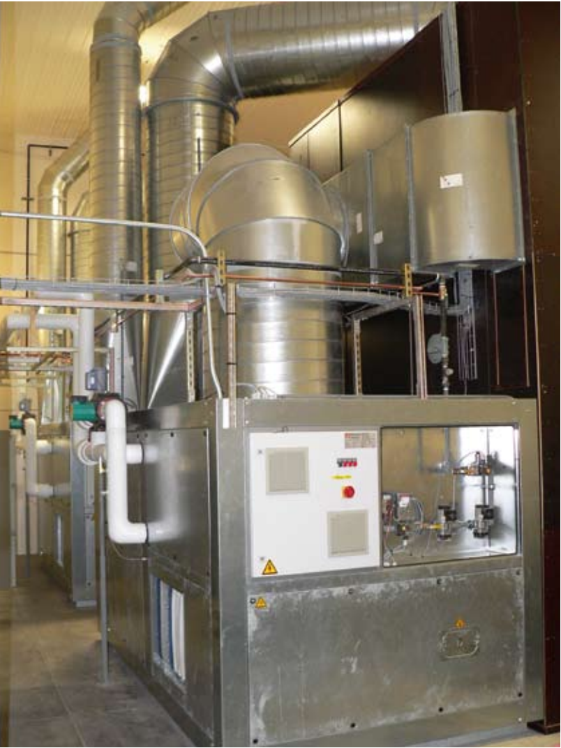
An absorption dryer reclaims energy by reusing warm and moist air to preheat incoming air flow
